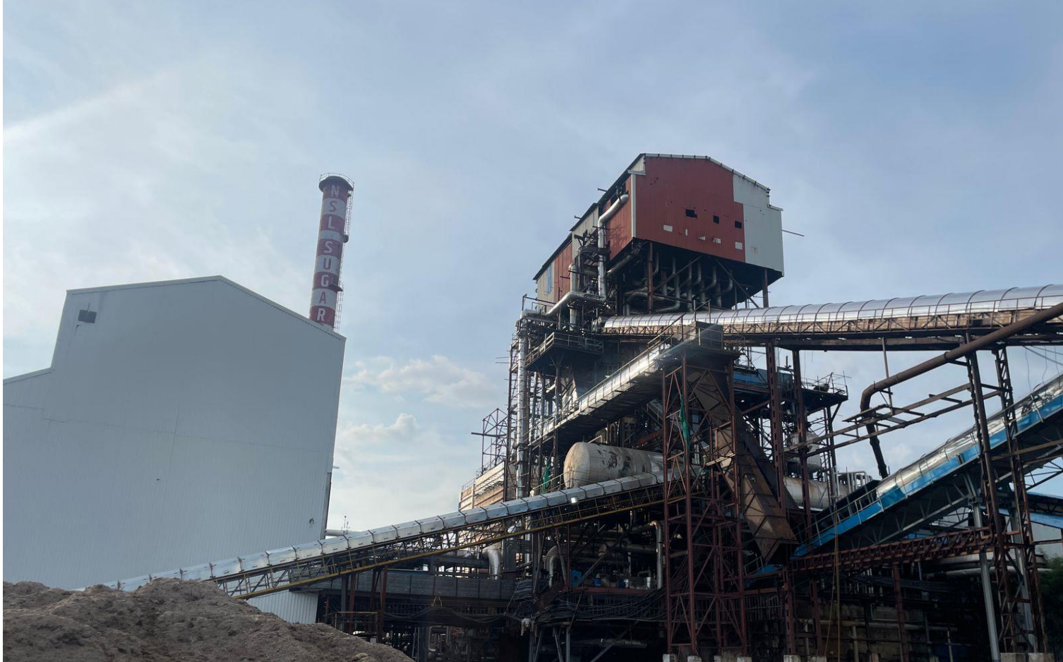
Picture 4: (a) Boiler house produce steam that's used in many stages of sugar manufacturing, (b) ESP, filtration device used in sugar factories to remove sugar dust and other fine particulate matter from a plant's flue gas stream
