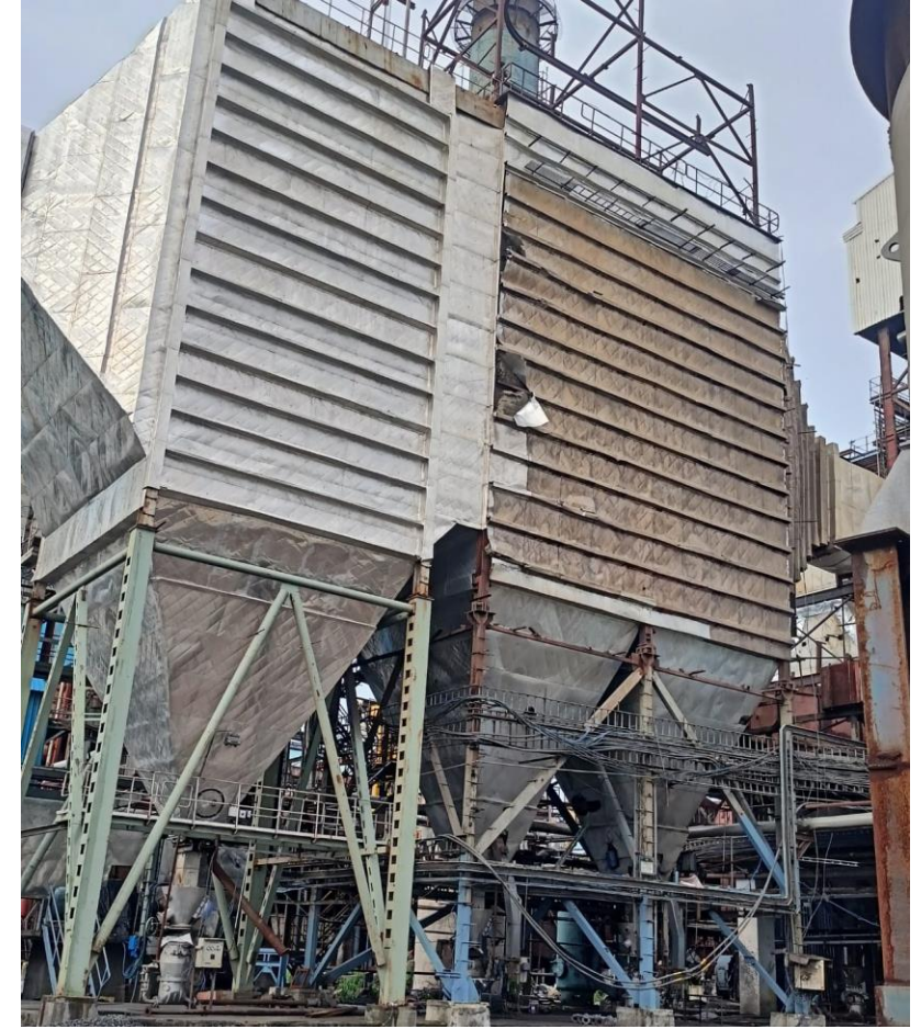
Picture 4: (a) Boiler house produce steam that's used in many stages of sugar manufacturing, (b) ESP, filtration device used in sugar factories to remove sugar dust and other fine particulate matter from a plant's flue gas stream
