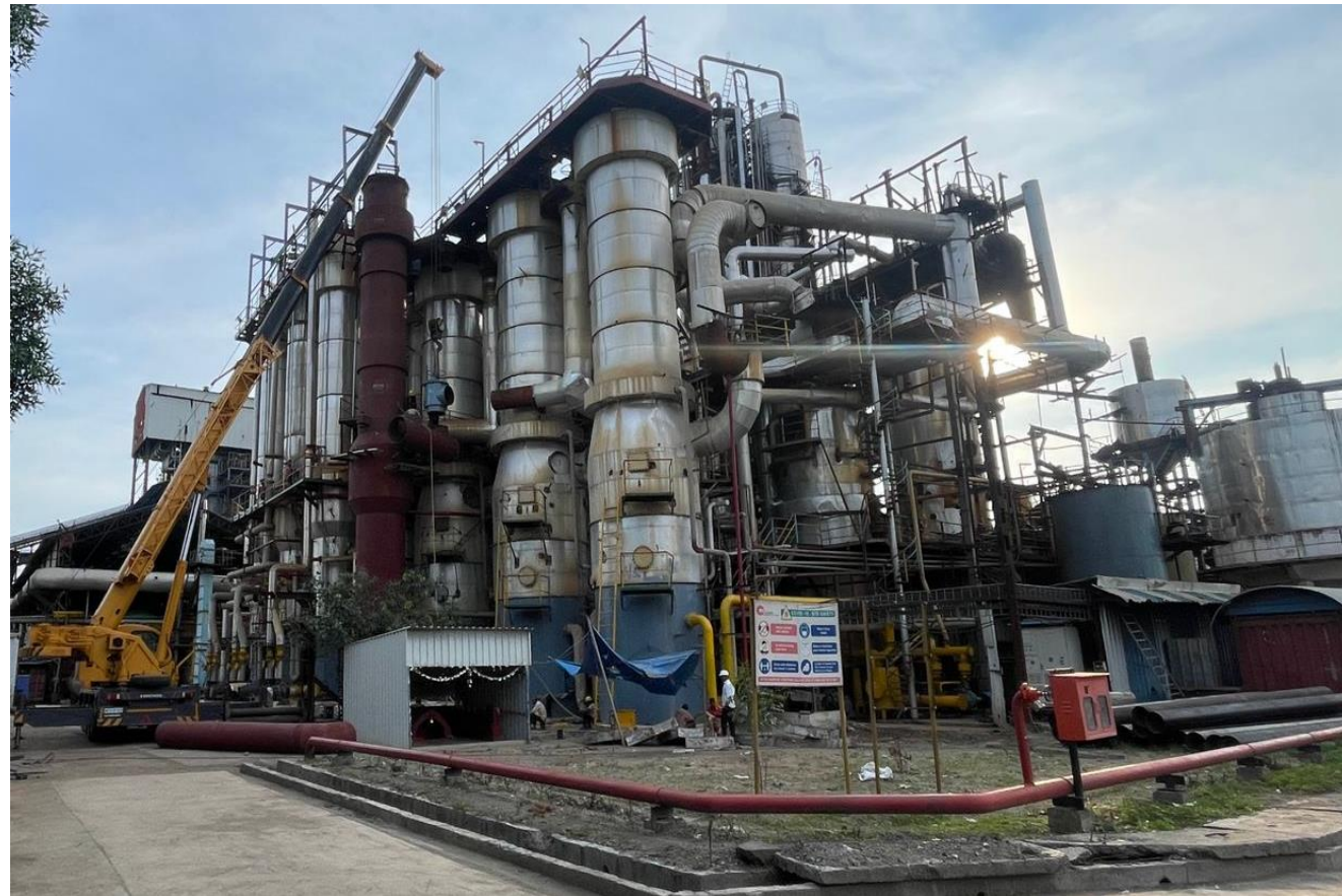
Picture 3: (a) Falling-film evaporators (FFEs) are used to concentrate juice through evaporation (b) Sugar house-processes sugarcane into sugar
