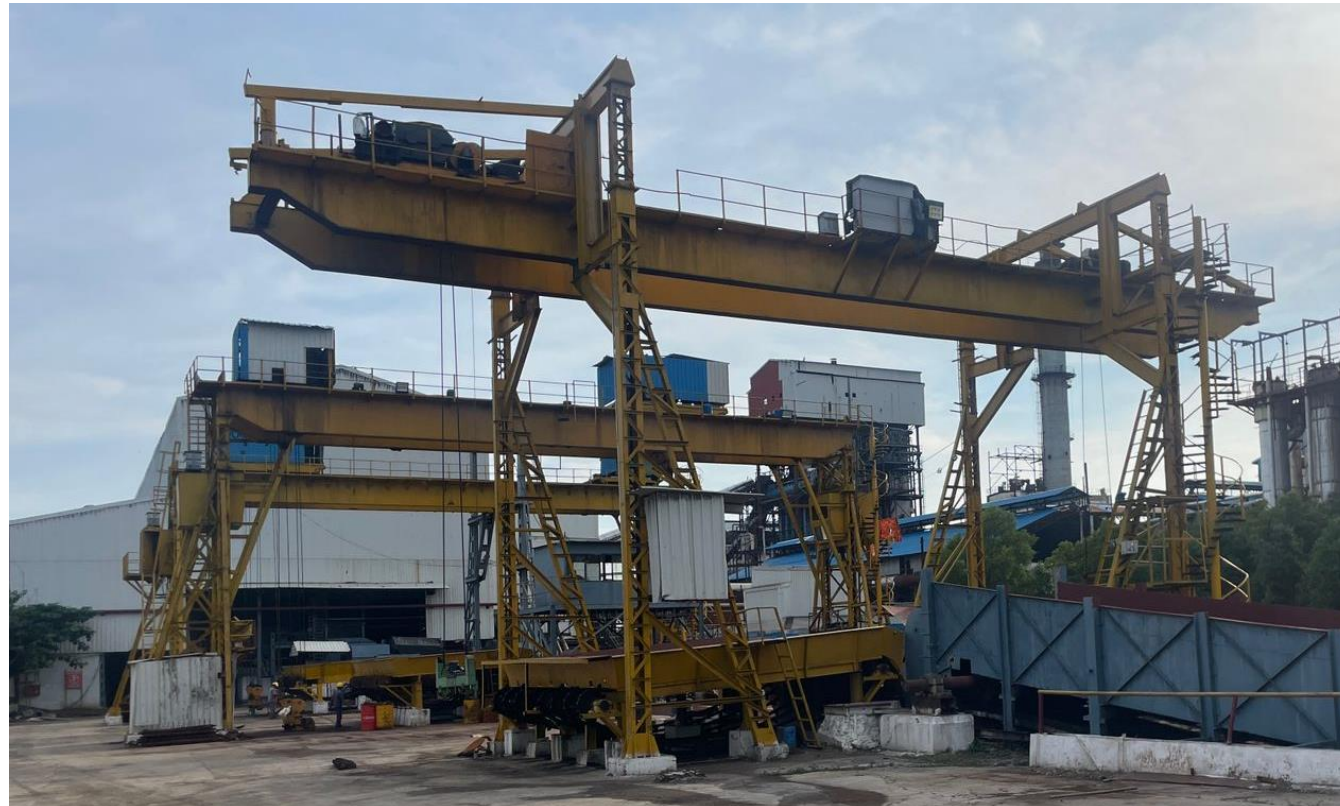
Picture 1: Cane carrier transports cane from the yard to the crusher
