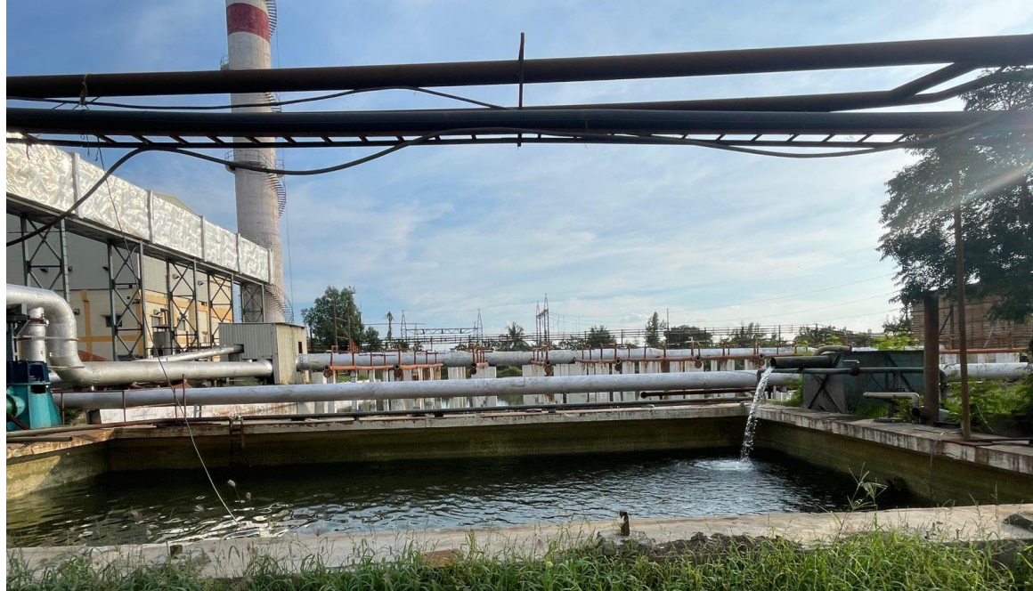
Picture 6: spray pond cools warm water from condensers and then pumps it back to the condensers and (b) Effluent treatment plant
